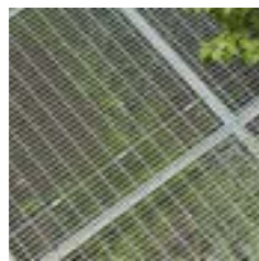
Galvanised Steel Walkway
