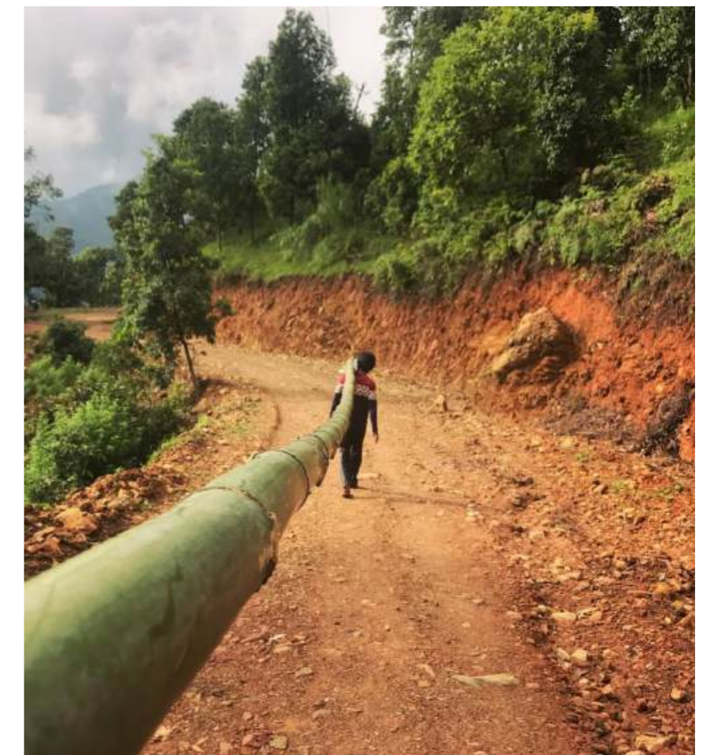
Building bamboo houses in Nepal
