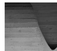
4. BOARD FORMED CONCRETE
