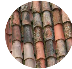
Reclaimed Roof Tiles
