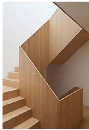
WOOD VENEER ENCASED STAIRCASE
