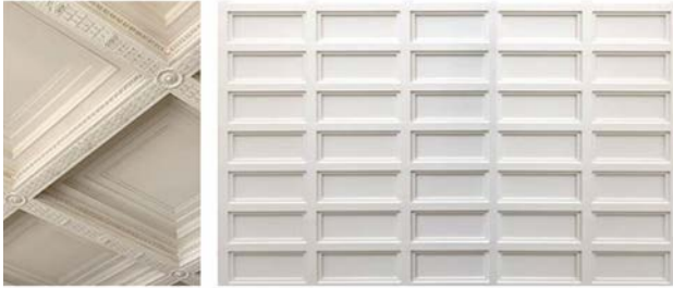
CEILING AND WALL PANELLING
